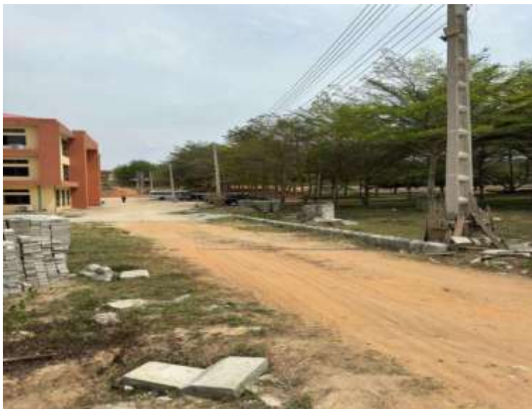
Plate 10: Unpaved zone beside academic building — bare laterite, stacked paving blocks awaiting installation
