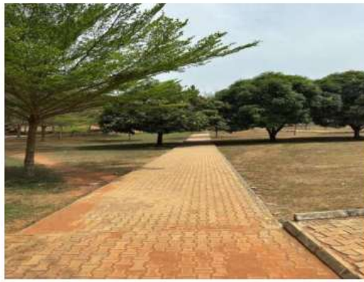
Plate 4: Secondary path through tree grove — partial shade, stained paving, absent edge definition
