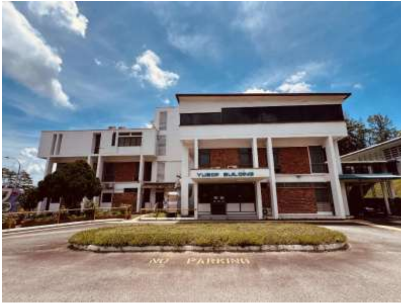
Fig 4.1.3: External view of SSVH showing building mass, façade treatment and window placement
